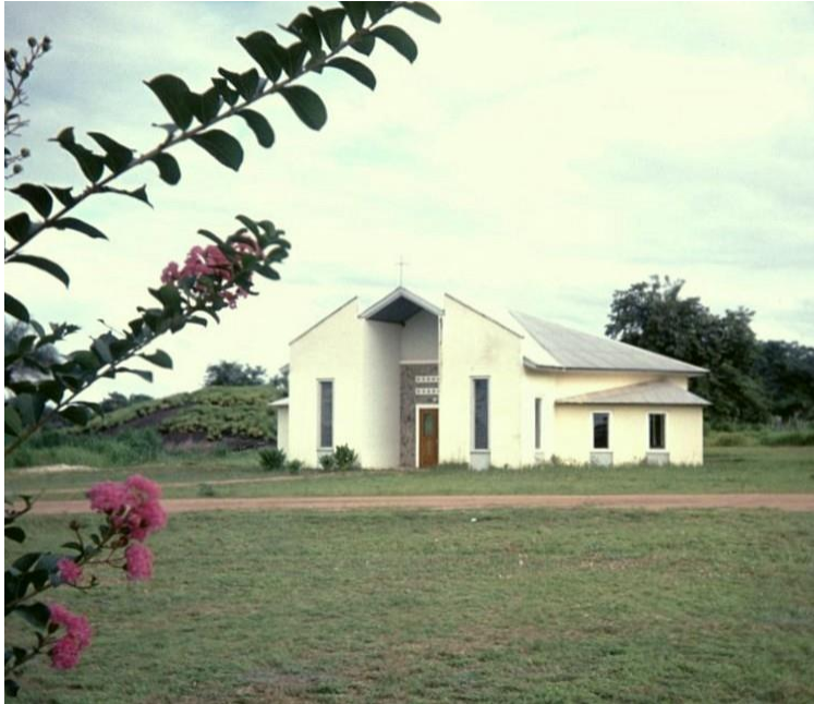
The Catholic Chapel at St Francis School
