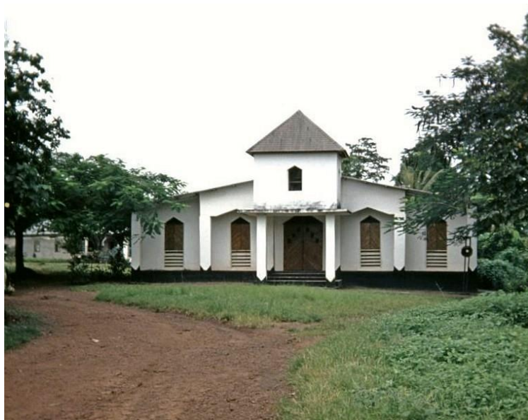
Kamakwie Methodist Church
