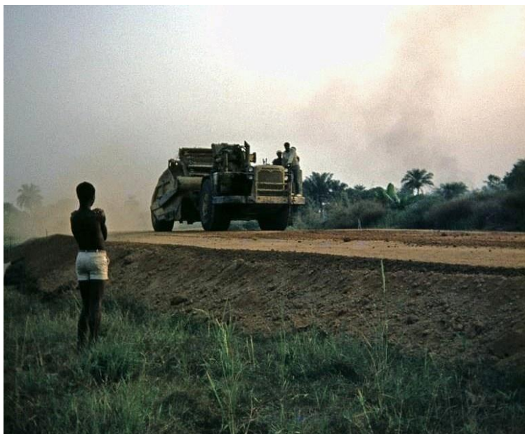
Heavy plant constructing the Makeni “by-pass”
