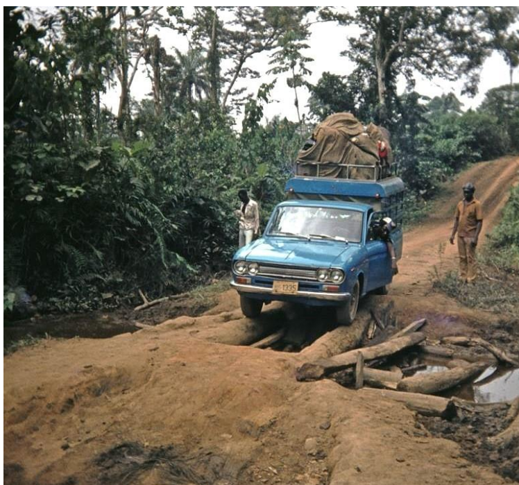
“Bridge” on the road from Sanniquellie to the Ivorian border
